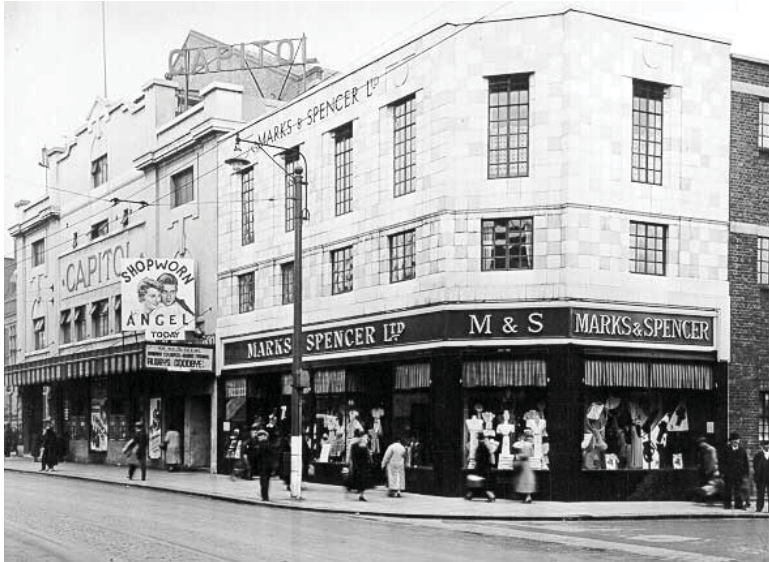
Figure 18 no.34 East Street circa 1935 when occupied by Marks and Spencers (source: Bird, E, (2007) Heritage Scoping study on Abbey and Barking Town Centre Conservation Area draft Design for London)
