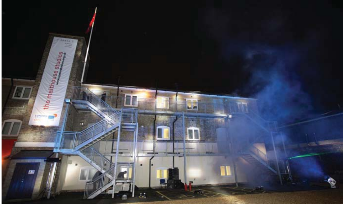
Figure 5 the Malthouse refurbished as part of the Creative Industries Quarter (source: LTGDC)
