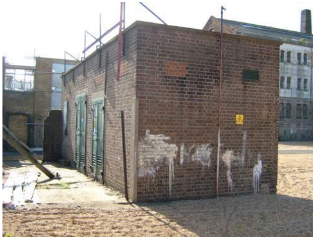
Figure 34 sub-station near the Abbey Road frontage (source: the writer)
