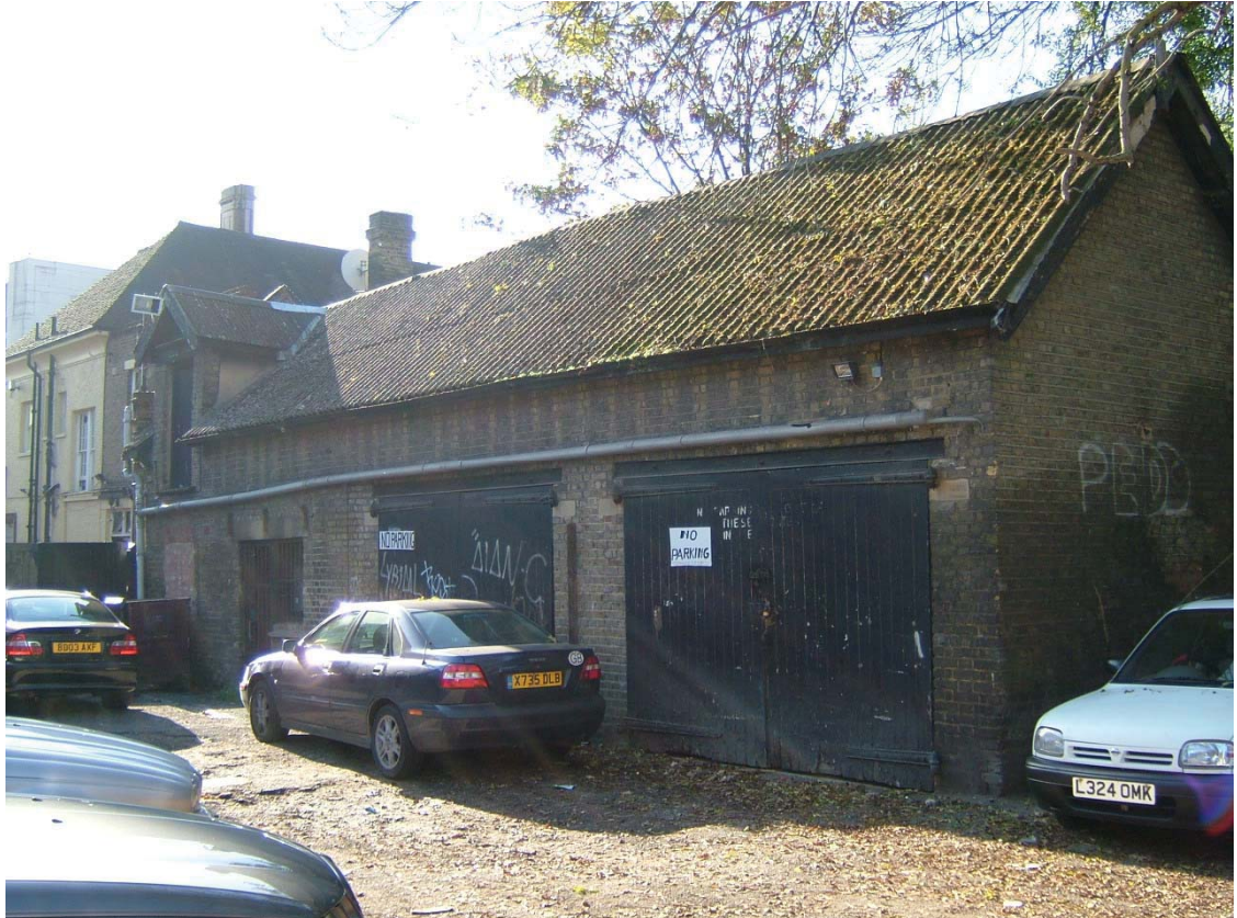
Figure 17 former stables complete with hayloft to rear of the Bull pub (source: the writer)
