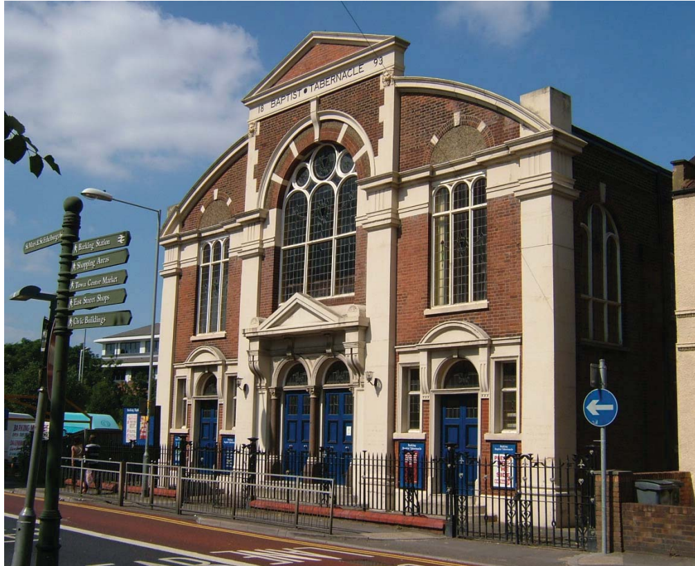
Figure 22 Renaissance style Baptist Tabernacle with its original features is a distinctive building on Linton Road (source: the writer)
