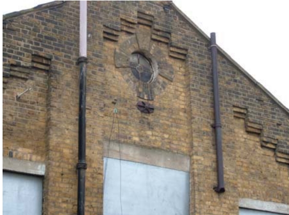
Figure 35 the gable ends now demolished which were on the Malthouse Extension (source: the writer)
