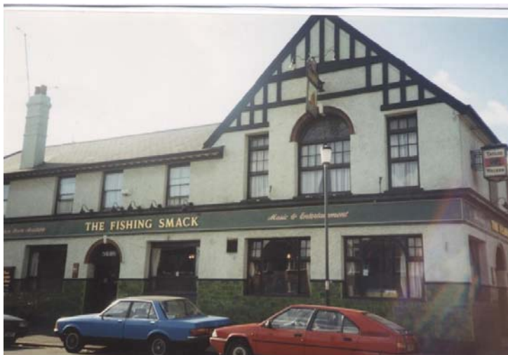
Figure 33 the Fishing Smack showing the rebuilt façade and extension (source: the writer)
