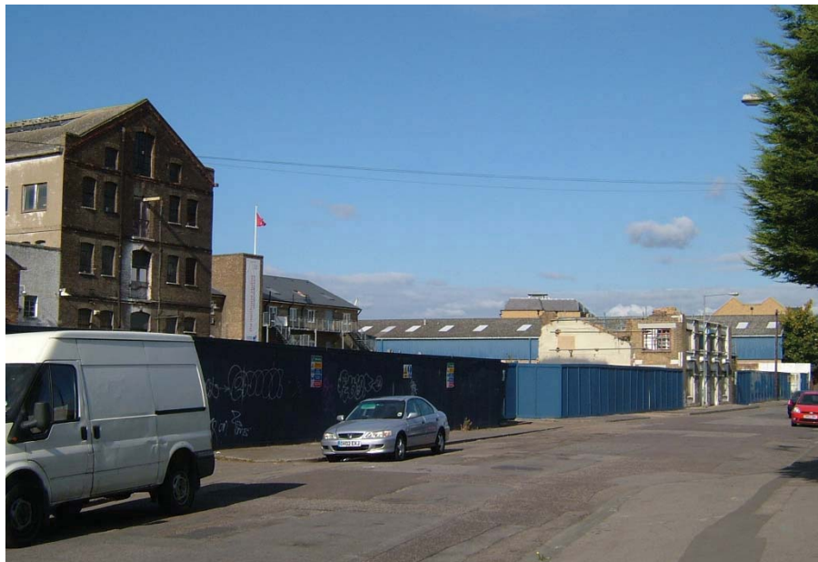
Figure 30 showing the façade of the barley loft on Abbey Road (source: the writer)
